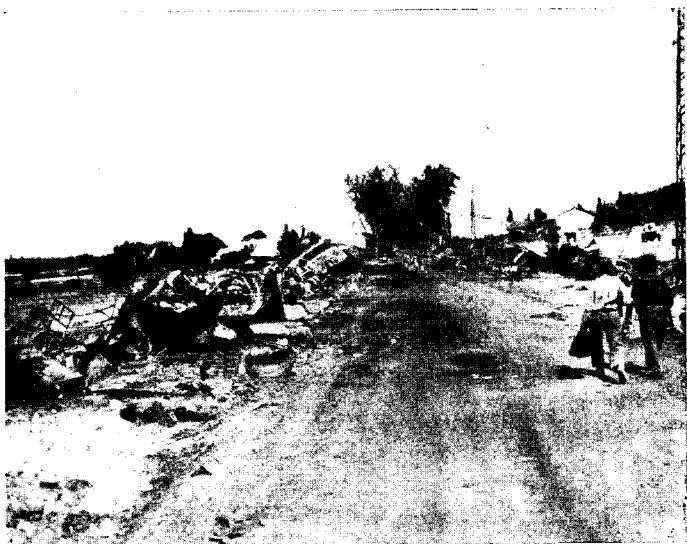
THE MONTELIMAR DESTRUCTION WAS COMPLETE
